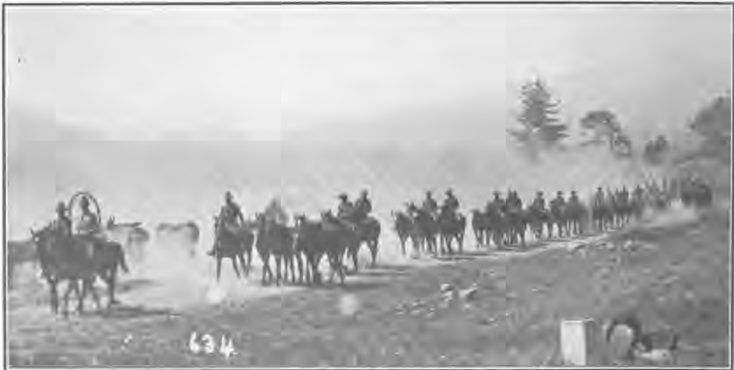
115TH ENGINEERS AT CUYAMACA LAKE.
